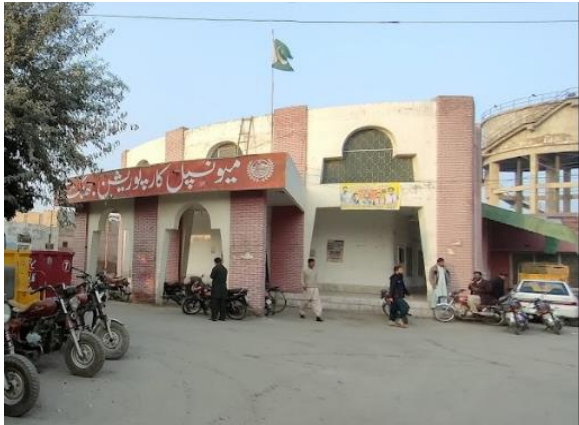
Figure 13: Front view of Main MC Building
