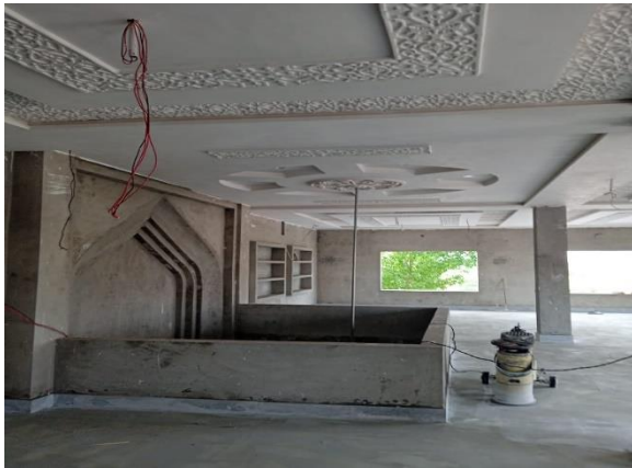
Figure 44: Front View Of Mosque
