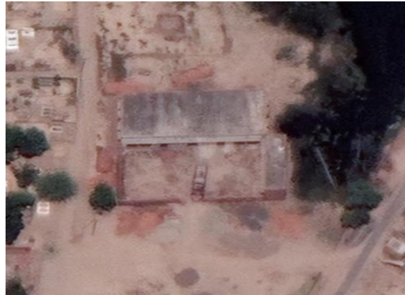
Figure 42: Aerial view of Graveyard
