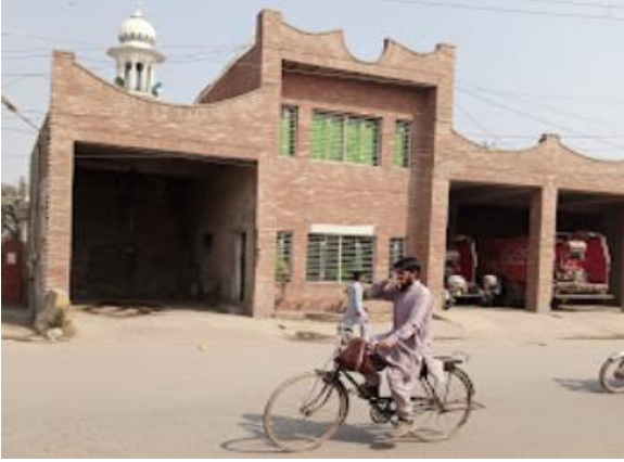
Figure 31: Front view of Fire Brigade
